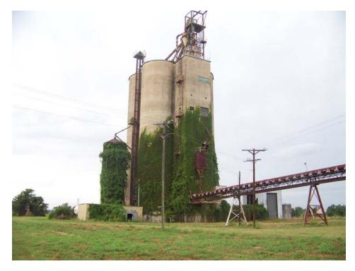
Photograph 1. Grain silo, showing flammable shed, shop, dryer on left, truck dump on right, and conveyor
