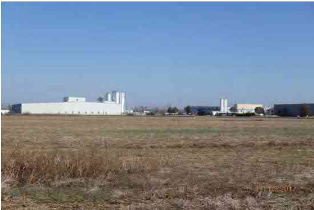
Adjacent industrial operations.
