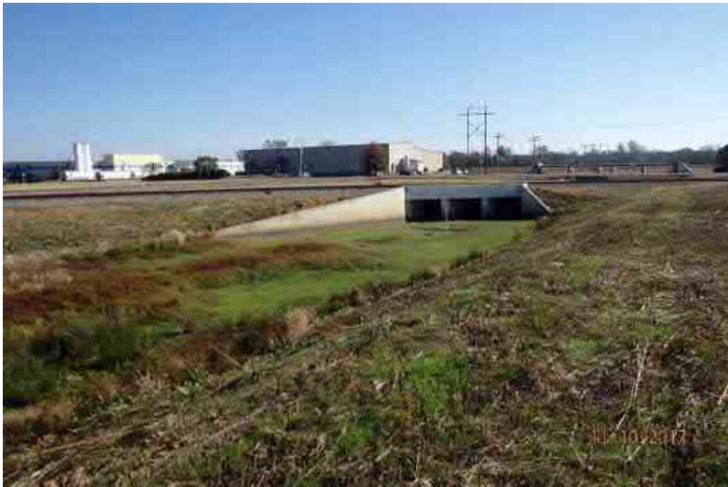
Drainage ditch at NE property boundary.
