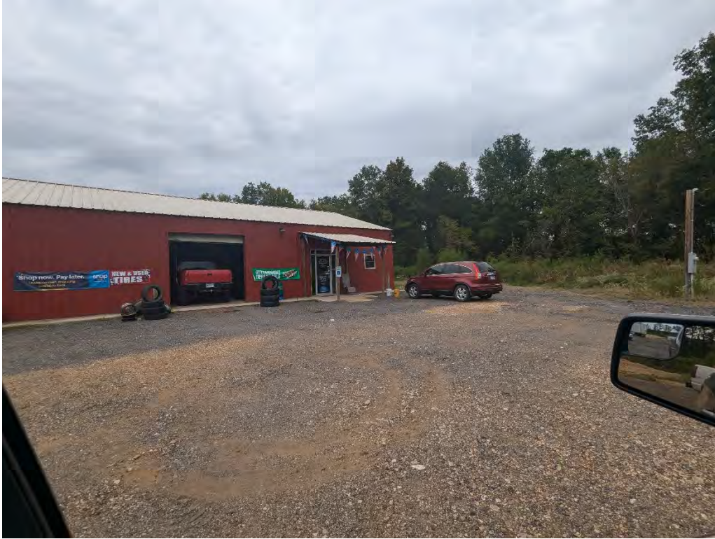
Photograph 31: Tire shop east of the subject property and west of Hwy 67.
