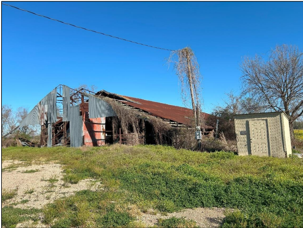
Figure 35. Barn and pump house, facing northwest.
