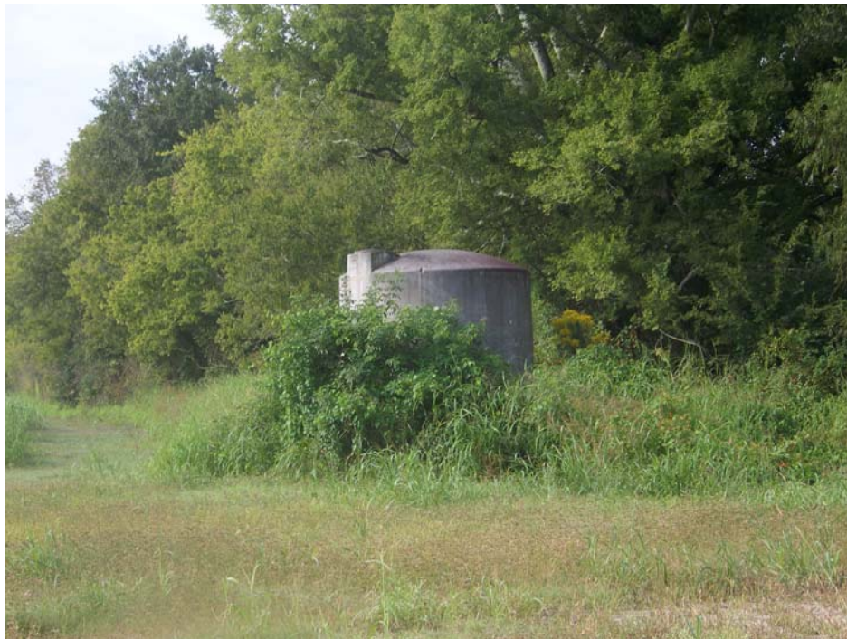
Photograph 8. Water storage tank near slabs in north central portion of property
