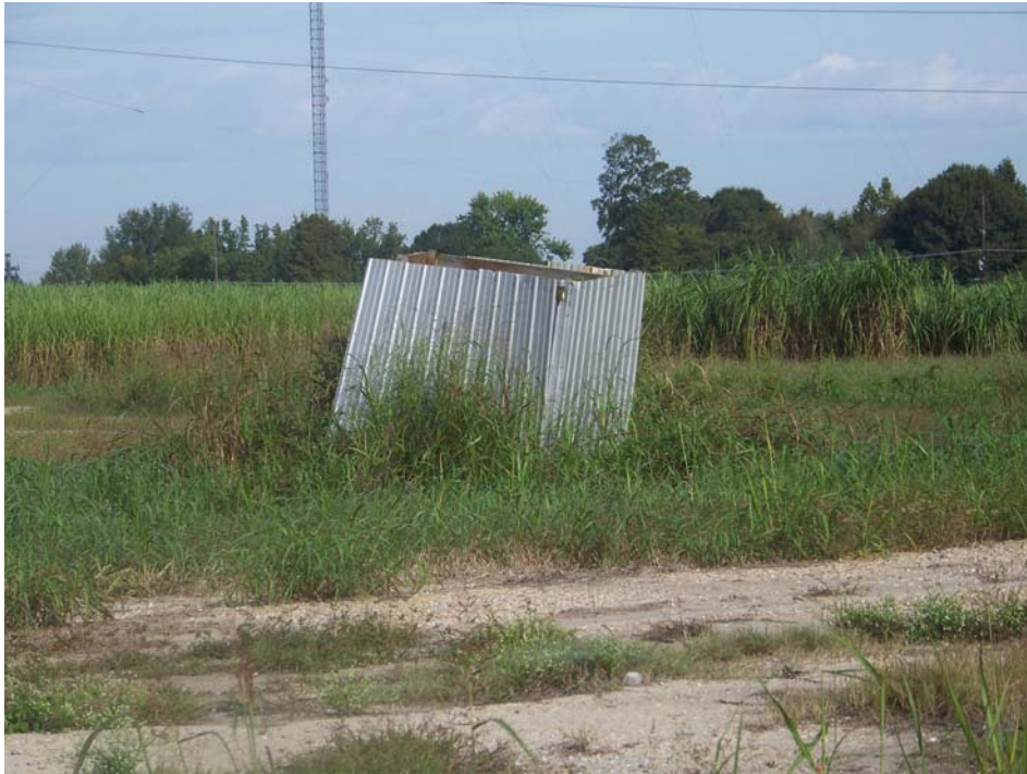
Photograph 7. Blown-over well shed near slabs in north central portion of property
