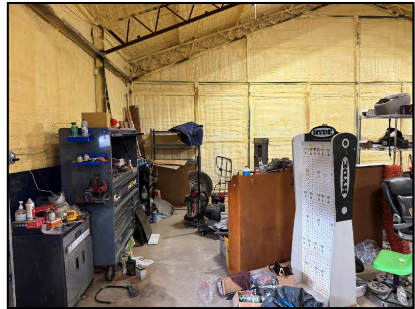
Photograph 6: Additional view of secondary room.
