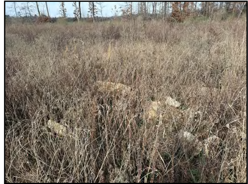
Photograph 20: View of discarded concrete located in western portion of property.
