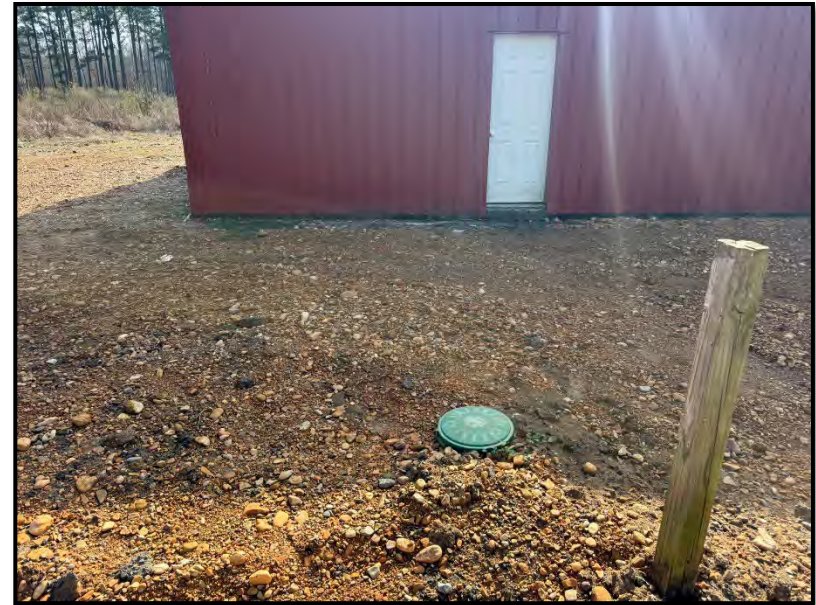
Photograph 18: View of septic system adjacent to western side of building.
