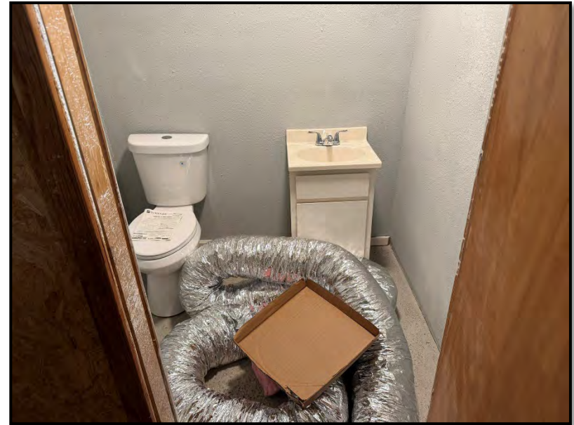
Photograph 10: View of additional restroom inside building.
