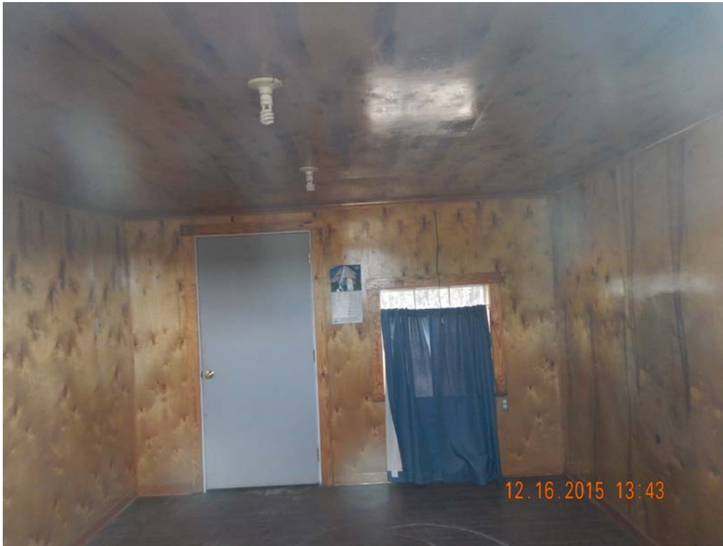
Photograph 17. View of south orchard building interior.
