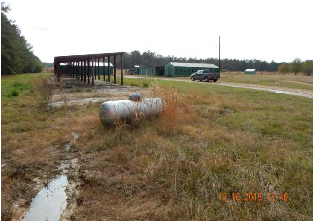
Photograph 13. Orchard structures viewed from north.
