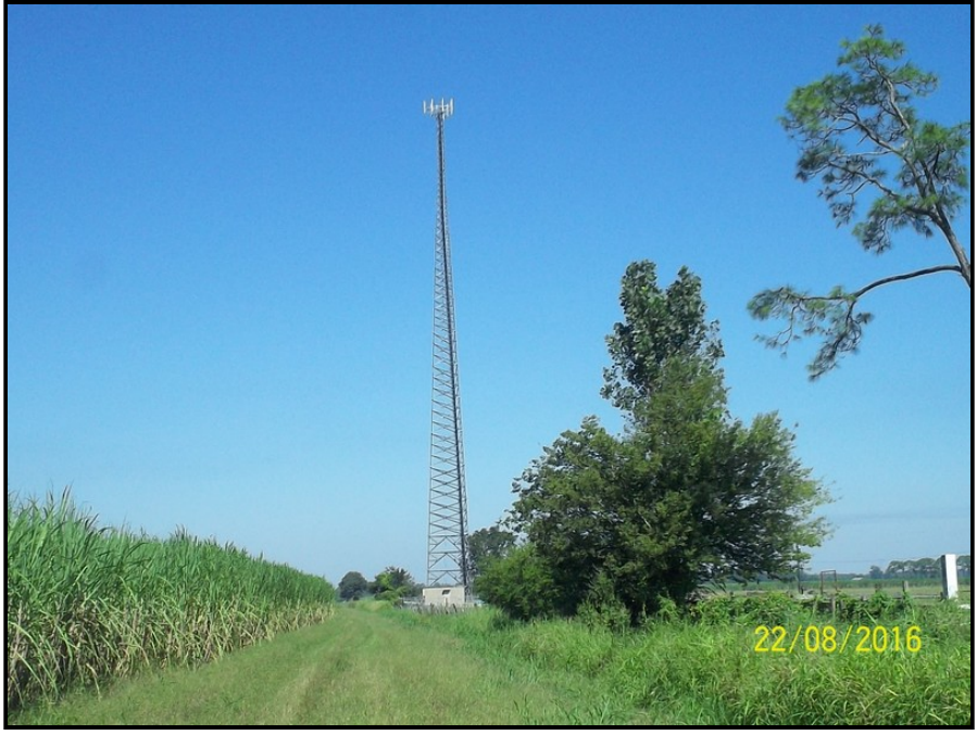
Photo 46: View of the cellular tower on the northeast adjoining property facing northwest.
