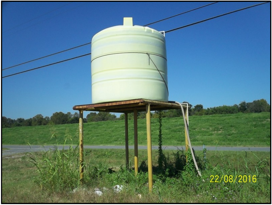
Photo 32: View of the water tank on the northwest portion of the subject property along Highway 405.
