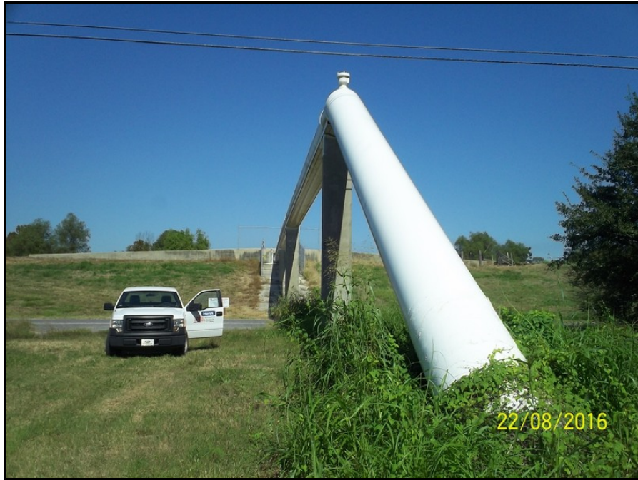
Photo 33: View of the waste water pipeline from the Mississippi River and over Highway 405 traversing along the northeast boundary of the subject property.
