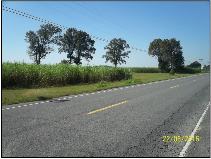
Photo 35: View of the north corner of the subject property from Highway 405 facing south.
