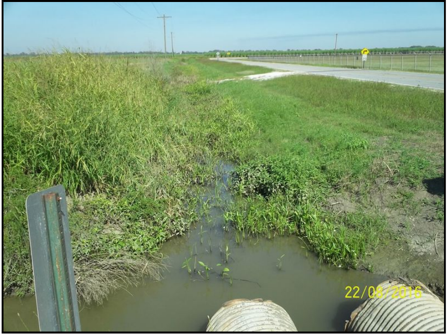
Photo 16: View of drainage feature on the subject property facing northwest.
