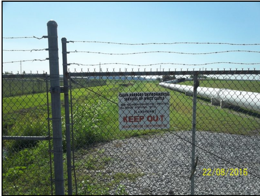
Photo 5: View of secured access gate to the Clean Harbors waste facility off Clark Road.
