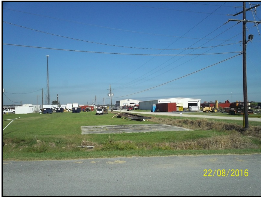
Photo 1: View of the Maintenance Enterprises facility located adjoining the east corner of the subject property.
