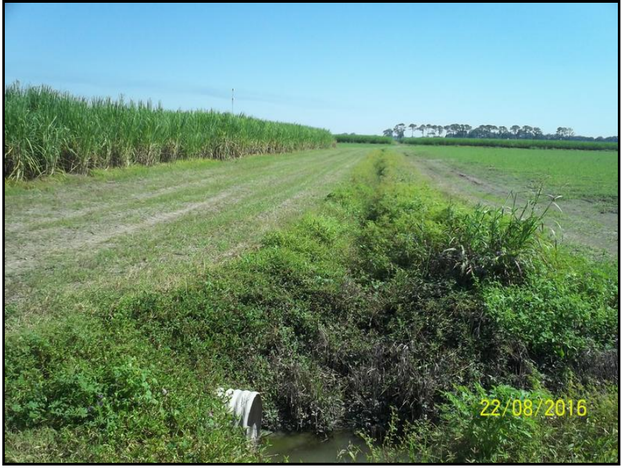
Photo 40: View of drainage features on the interior of the subject property facing northeast.
