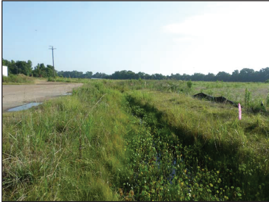
Wet Ditch facing North
