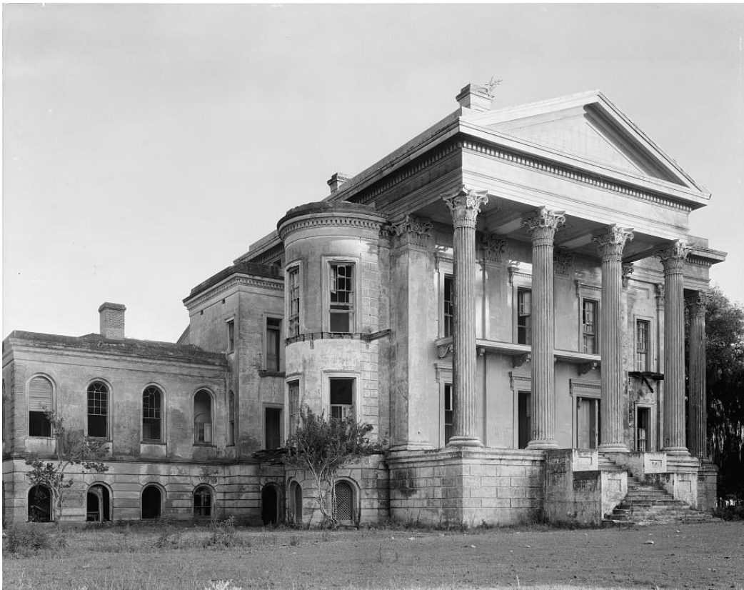
FIGURE 15. FRONT (RIVER FACADE) OF BELLE GROVE PLANTATION BIG HOUSE 1938 (SOURCE: LIBRARY OF CONGRESS).
