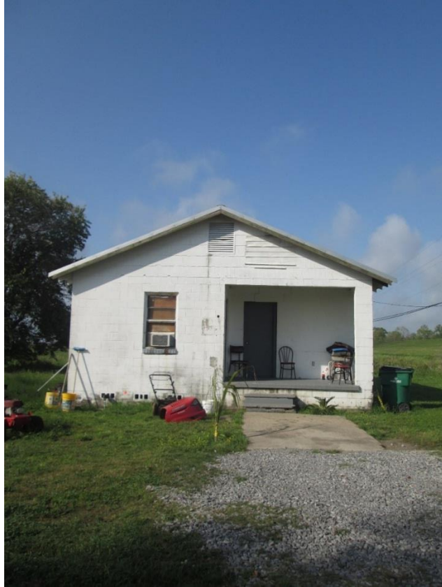
FIGURE 40. STANDING STRUCTURE, NORTHEASTERN WALL; FACING SOUTHWEST.
