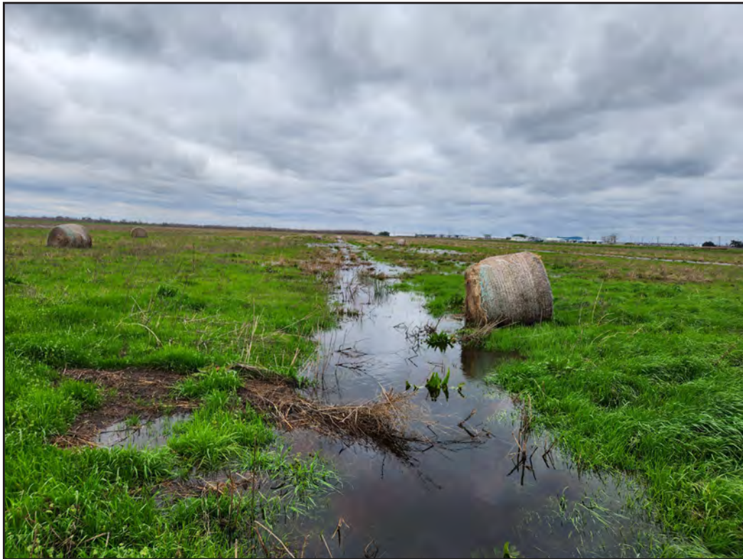
Figure 5.3. View of the eastern drainage ditch in the north portion of the project area, facing north.
