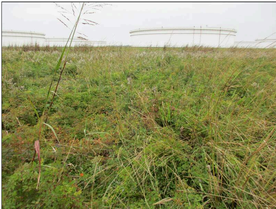
18 - Overview of DP4, facing east.
