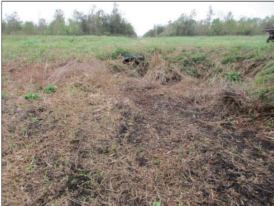
28 - Overview of confluence of S3 and S1, facing south toward culvert.
