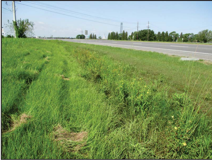
Photo 39: Appearance of the drainage ditch traversing along Highway 70.
