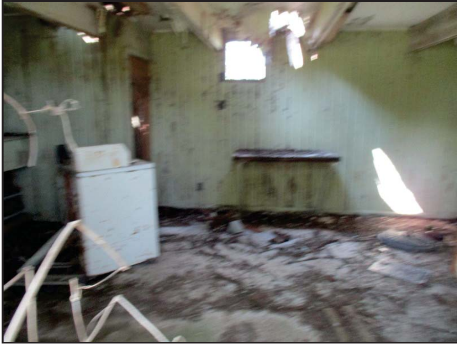
Photo 41: Appearance of the inside of the wooden building.
