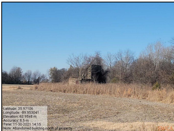
Photo 17: Abandoned skeet range building northwest of subject property, facing northwest.
