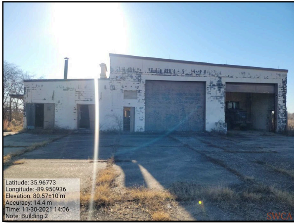
Photo 13: Facade of building #2, facing southwest.
