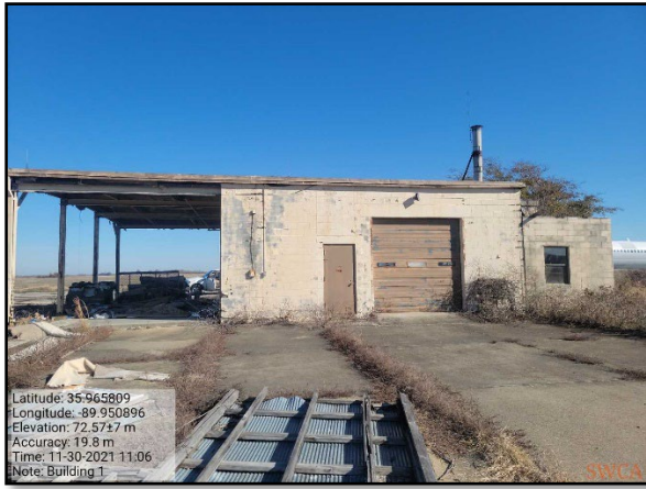
Photo 1: Facade of building #1, facing northeast.
