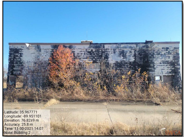
Photo 14: Facade of building #2, facing southeast.
