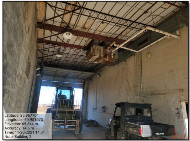
Photo 8: Interior of garage in building #2.
