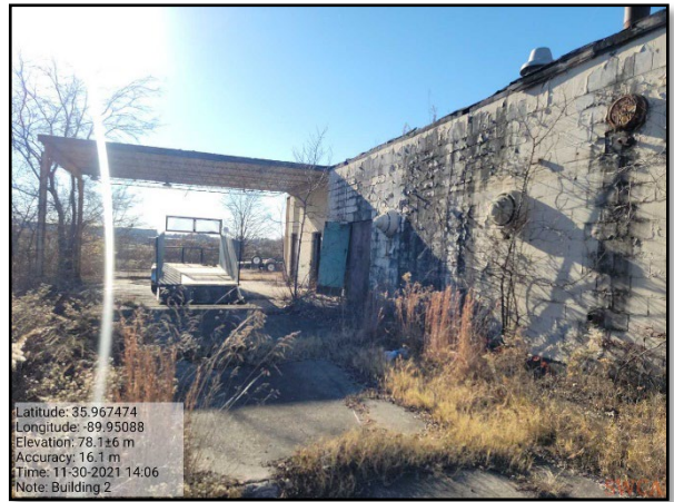
Photo 12: Facade of building #2, facing southwest.
