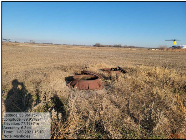
Photo 21: Manholes on subject property, facing southeast.
