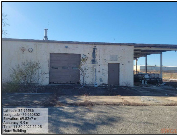
Photo 3: Facade of building #1, facing southwest
