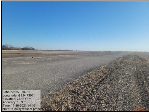
Photo 19: Airport runway exiting subject property, facing west.
