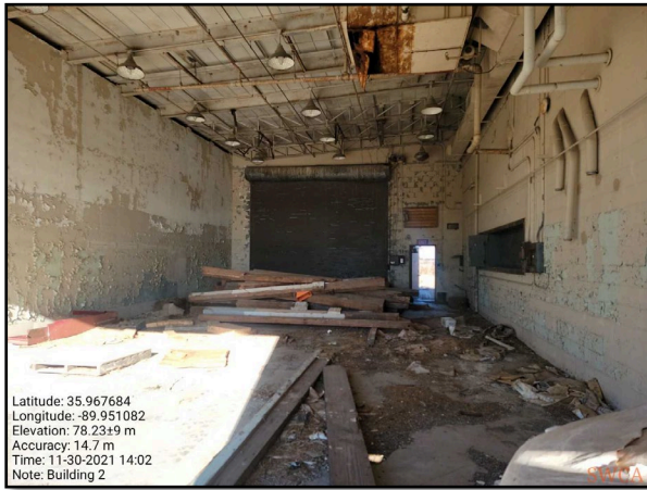
Photo 9: Interior of garage in building #2.
