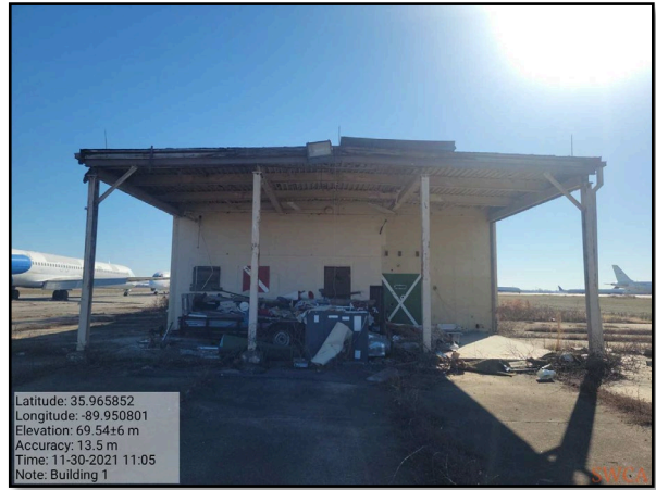
Photo 2: Facade of building #1, facing southeast.
