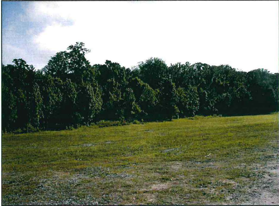
Figure 7. Overview photograph of the proposed power generation facility, facing northeast from southwest corner.
