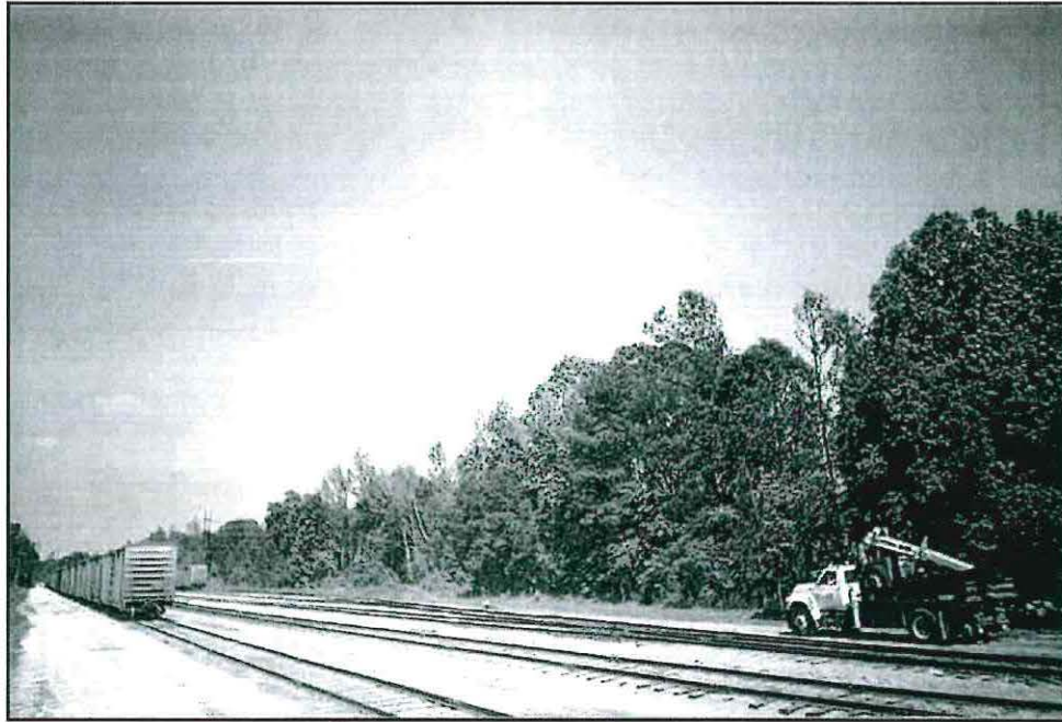
Figure 10. Overview photograph of the proposed power substation facility and transmission line corridor facing northeast.
