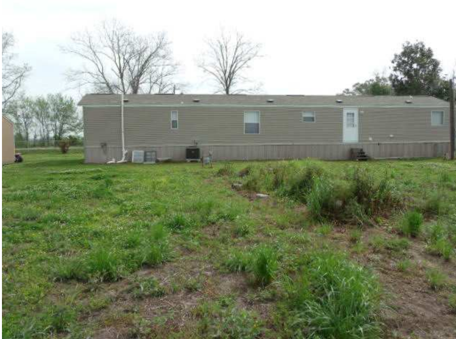
Figure 25. Backyard of trailer at 16IV55, showing utility meter; facing ENE.
