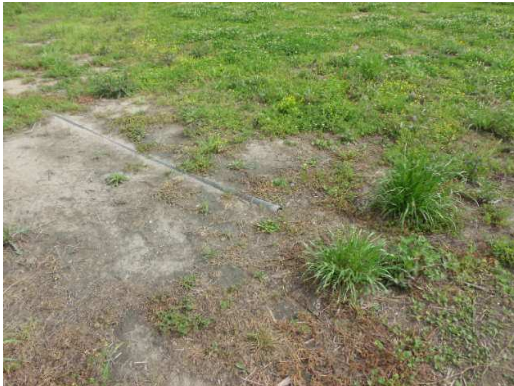
Figure 26. Pipe in backyard of trailer at 16IV55, facing NNE.
