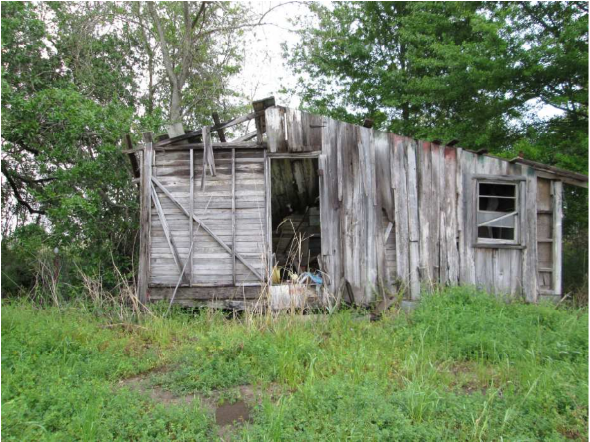
Figure 20. Abandoned outbuilding, north part of 16IV55, facing east.
