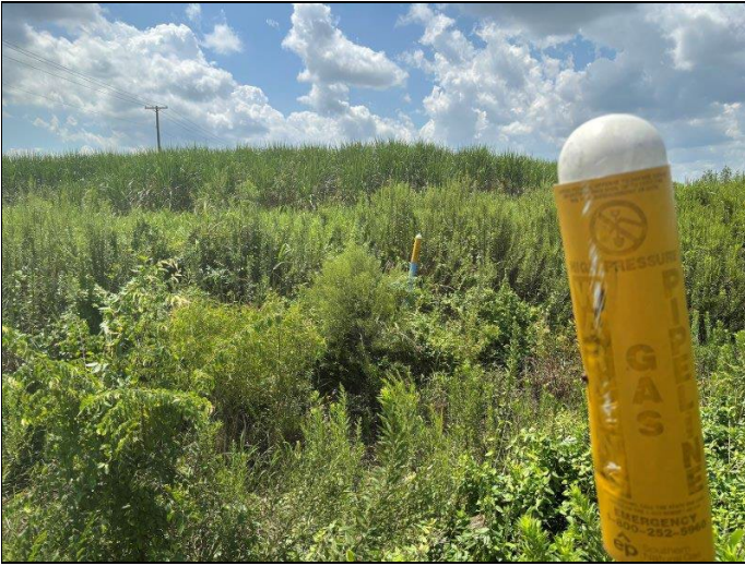
13. Natural gas pipeline marker in the southern part of the property
