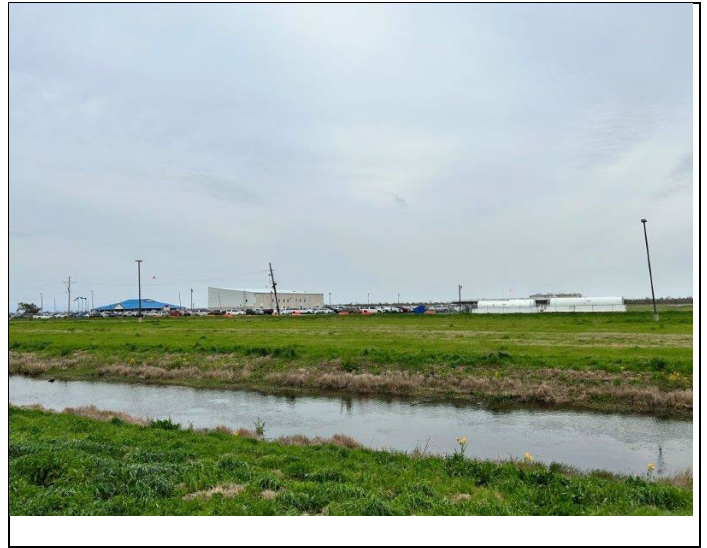
10. Bristow US LLC, SAR Center with two fuel tanks (east adjoining)
