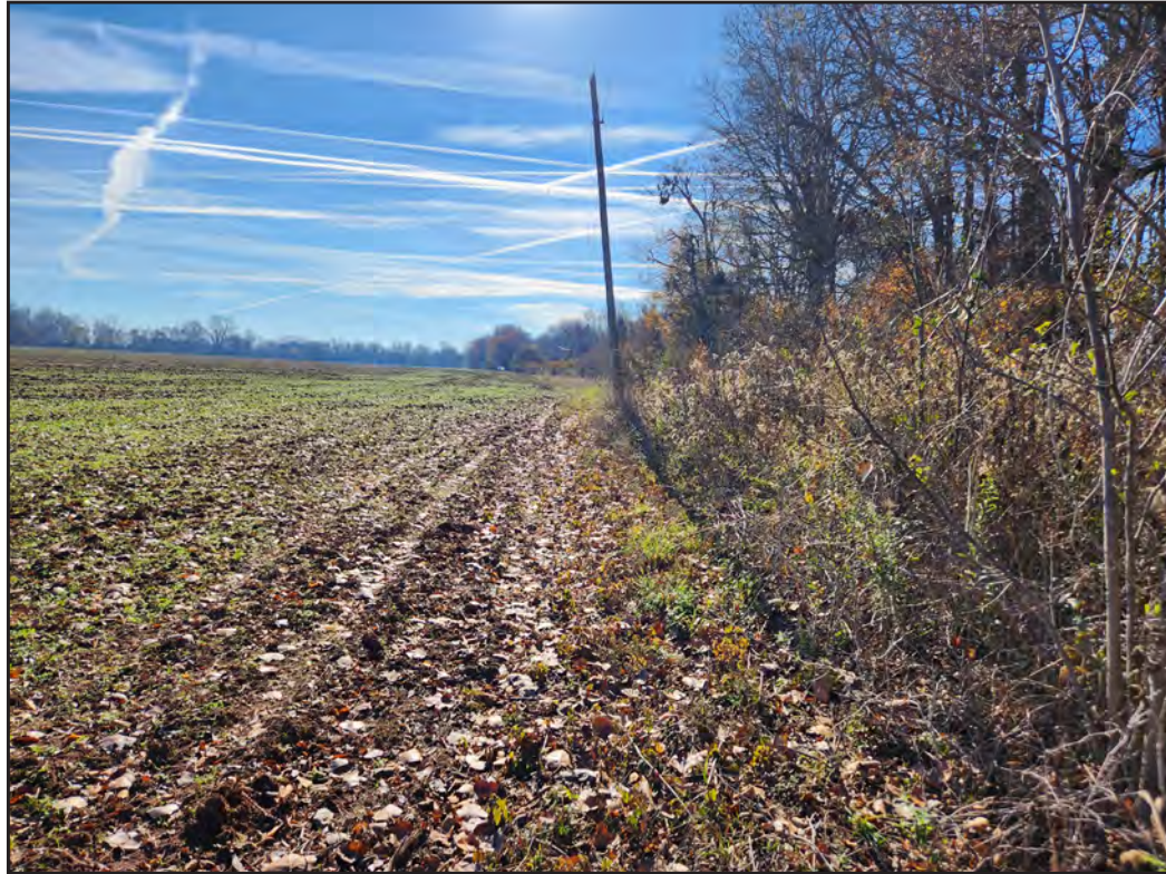
Figure 5.10. View of the overhead power line on the west side of the project area, facing south.
