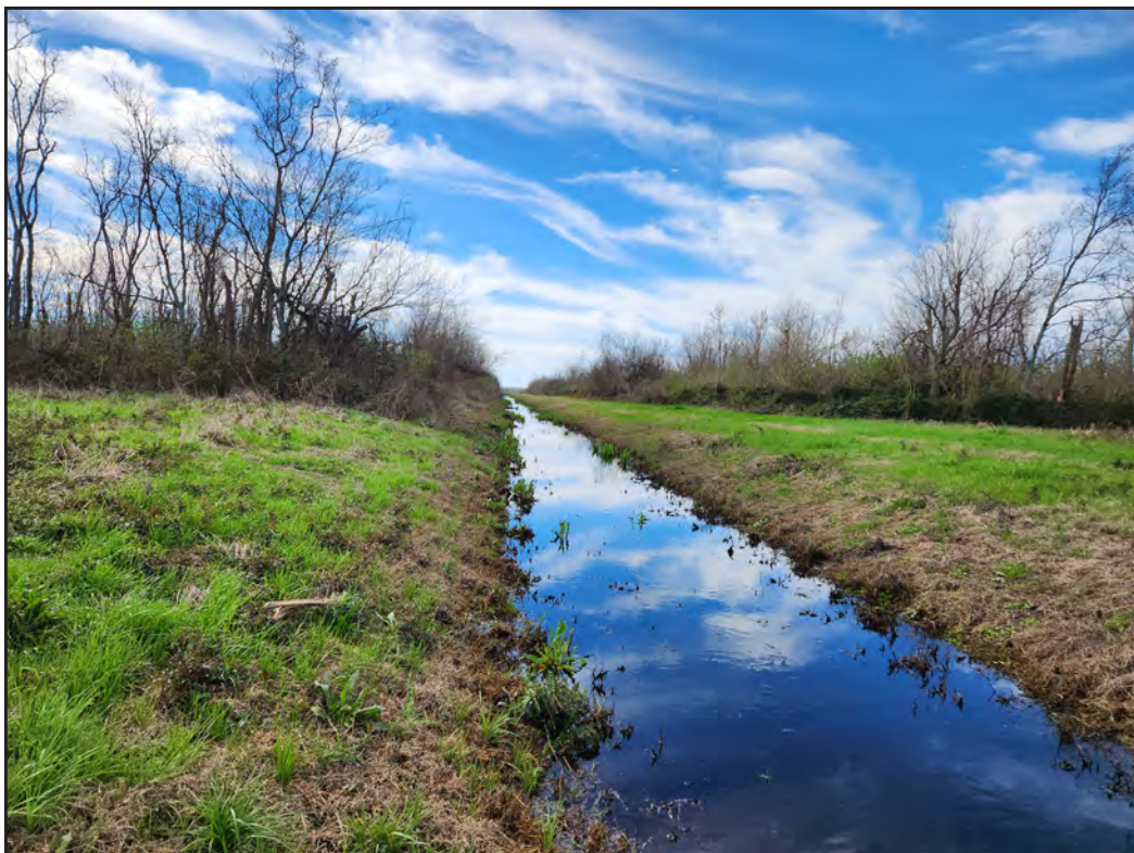
Figure 5.4. View of the drainage on the west boundary of the project area, facing south.
