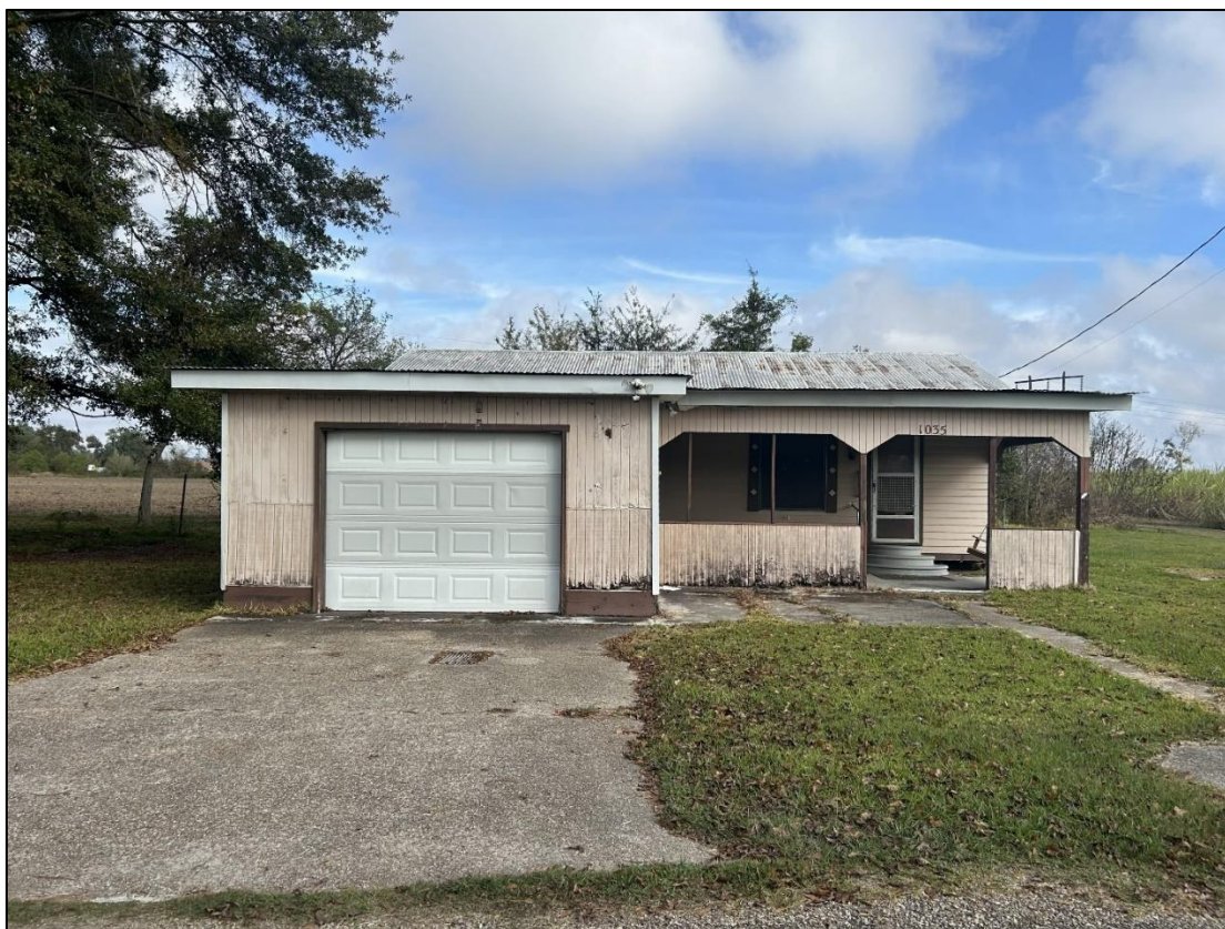
Figure 54. House at 1035 Ameda Berard Rd., facing north. (Resource No. 50-00804)
