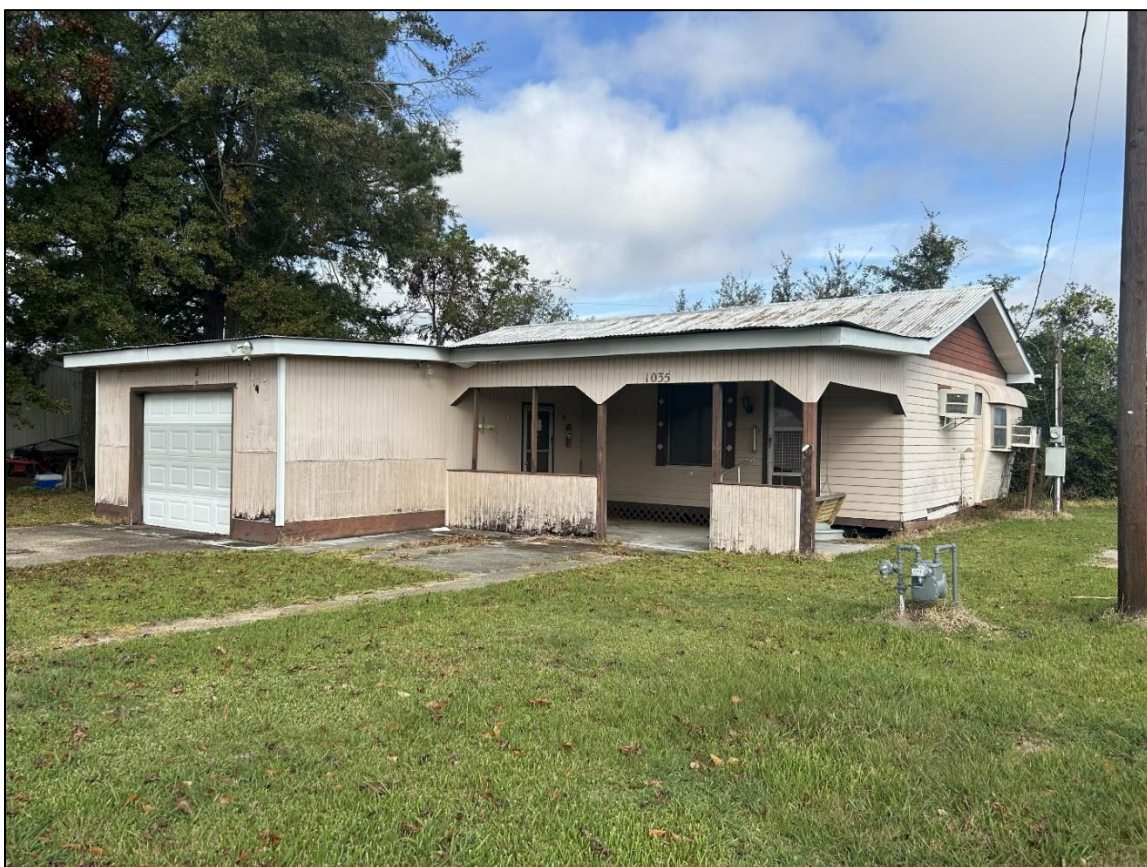
Figure 55. House at 1035 Ameda Berard Rd., facing northwest. (Resource No. 50-00804)
