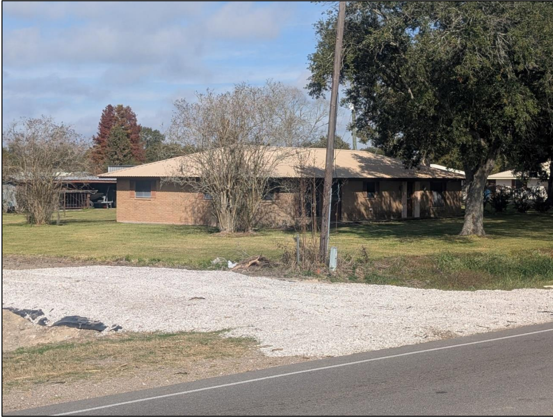
Figure 71. Structure at 2876 Grand Point Hwy, facing northwest.
