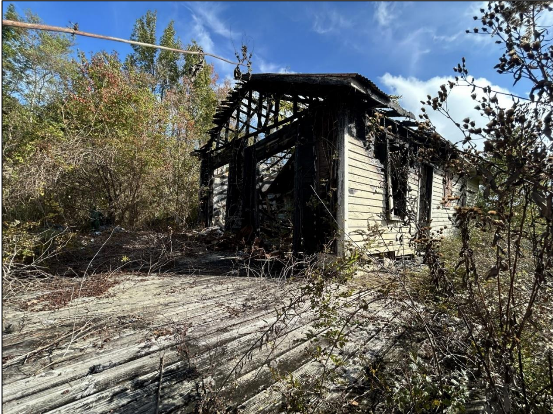
Figure 75. Building at 2894 Grand Point Hwy, facing northeast.
