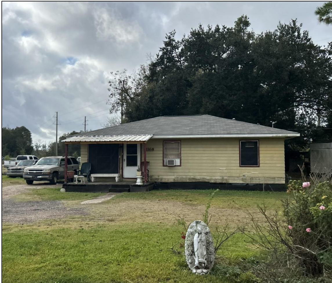
Figure 58. House at 1168 Melvin Dupuis Rd, facing southwest.
