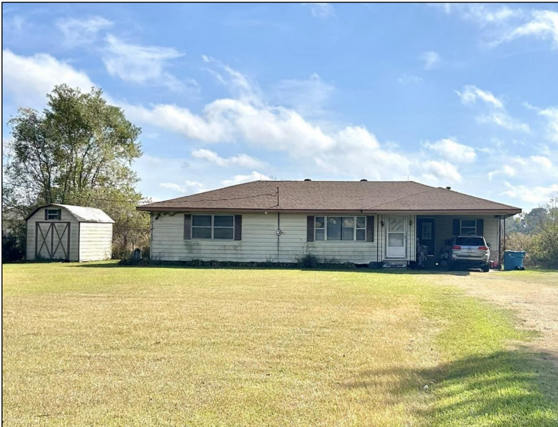
Figure 72. Structure at 2877 Grand Point Hwy, facing east.
