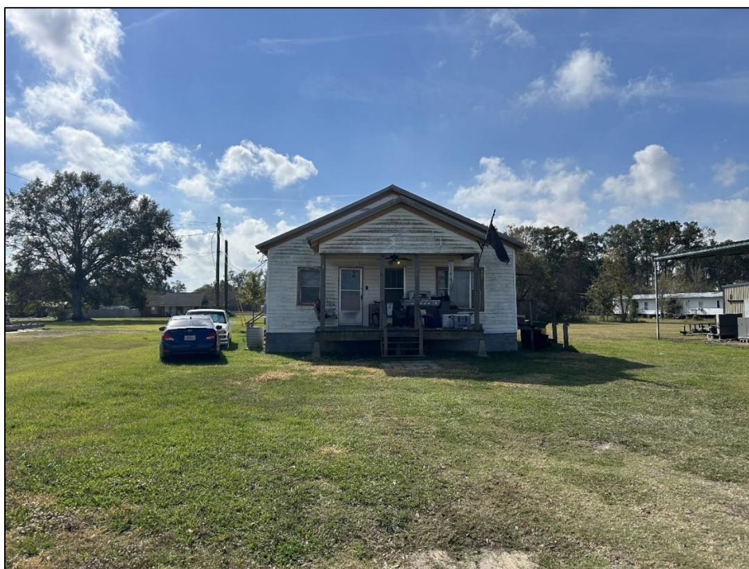
Figure 62. House at 1276 Dermelie Callais, Facing south.
