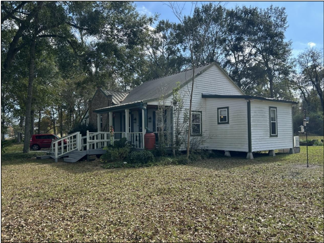
Figure 77. Structure at 1028 Shady Oaks Dr., facing northeast.
