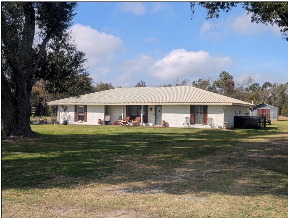
Figure 68. House at 2868 Grand Point Hwy, facing southwest.
