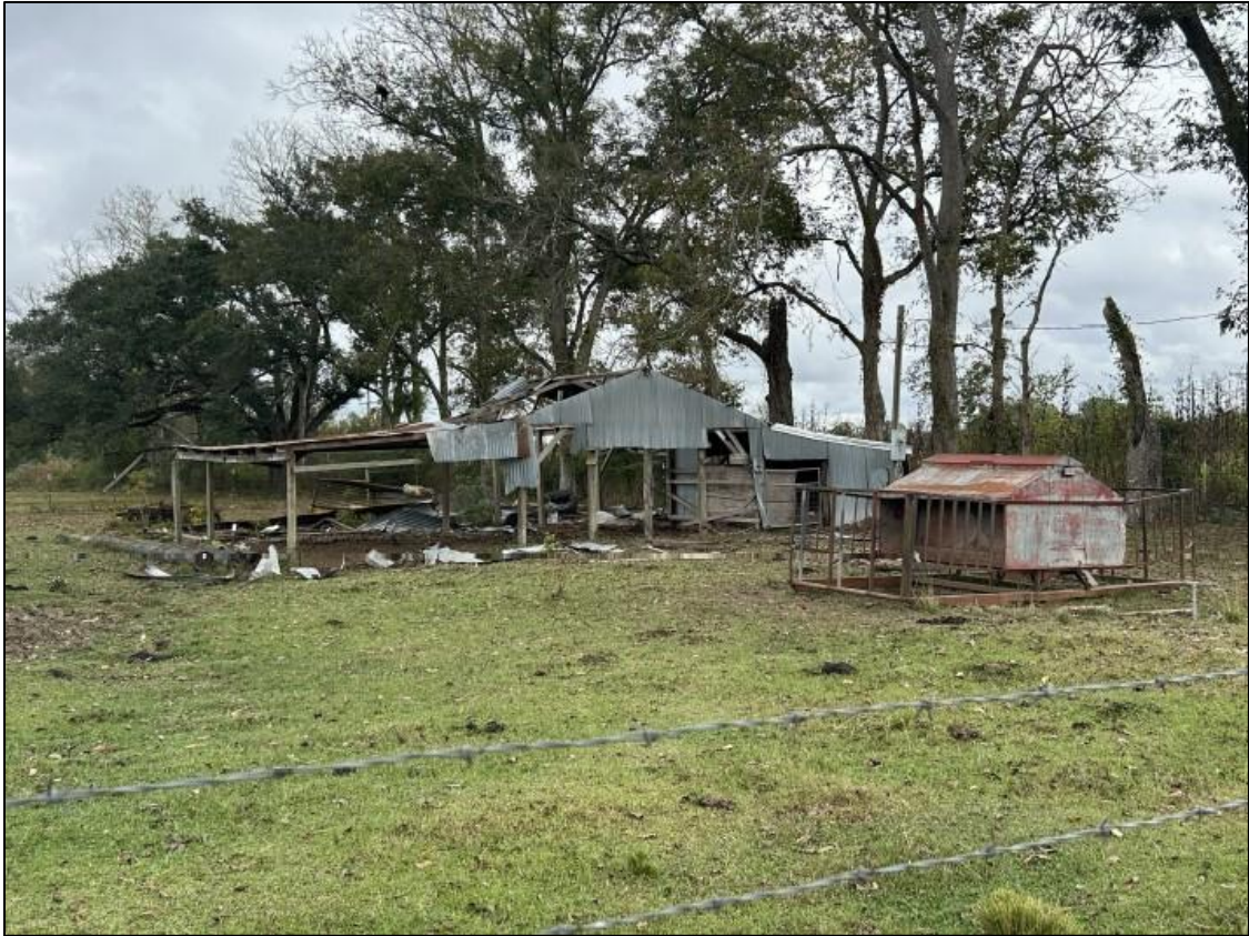
Figure 61. Barn off Melvin Dupuis Rd., facing northeast.
