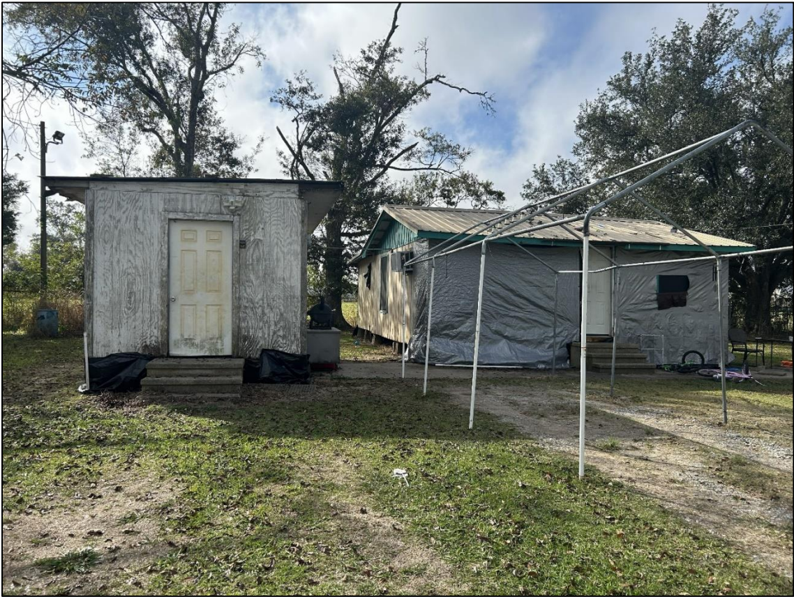
Figure 53. Structures at 1028 Ameda Berard, looking south. (Resource No. 50-00803)
