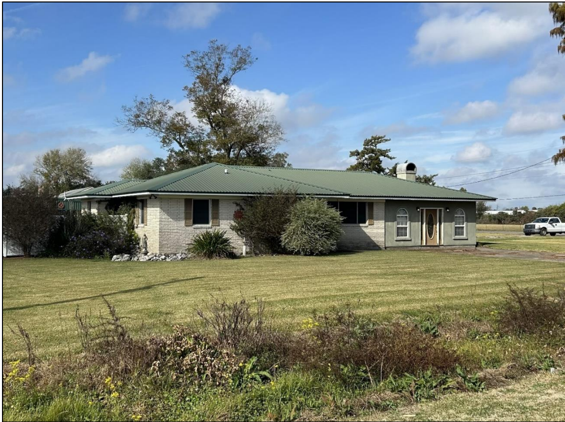
Figure 64. 2838 Grand Point Hwy, facing northwest.
