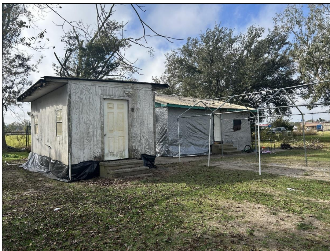
Figure 52. Structure and outbuilding at 1028 Ameda Berard, looking southwest. (Resource No. 50-00803)
