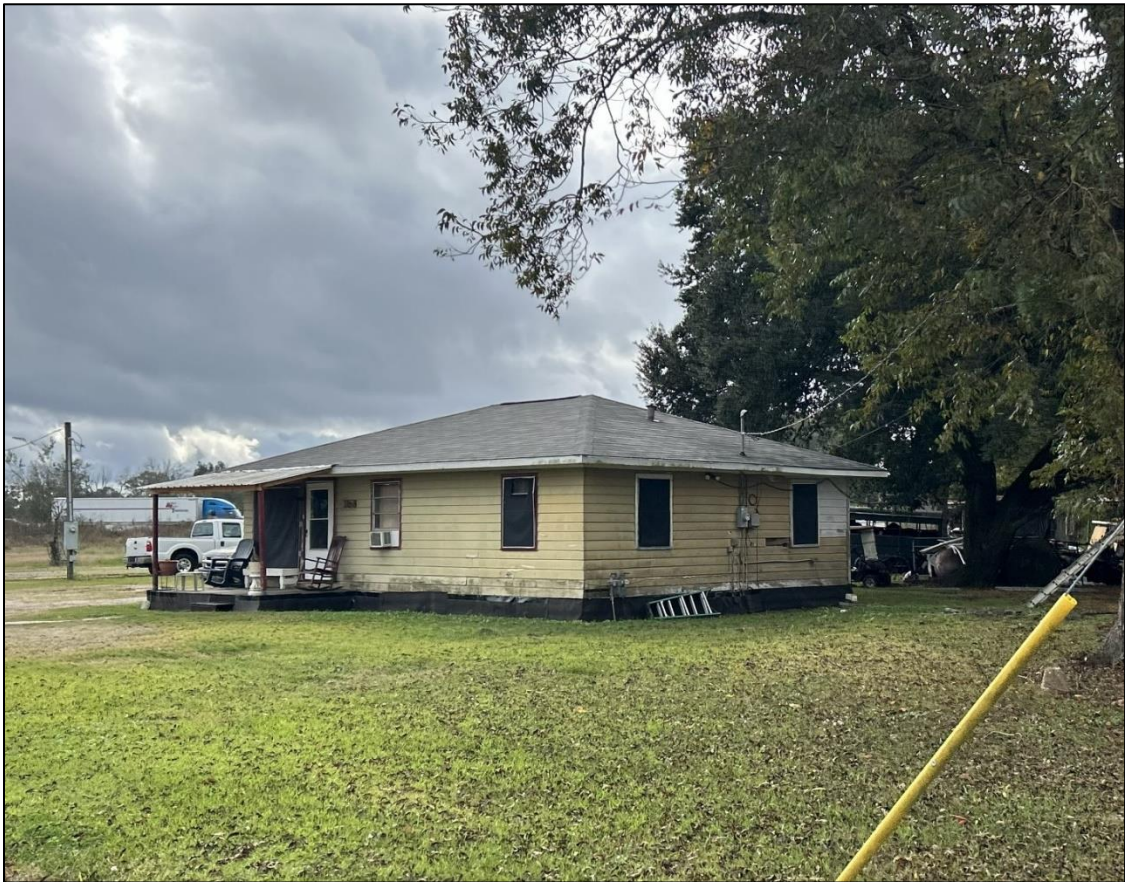
Figure 59. House at 1168 Melvin Dupuis Rd, facing south.
