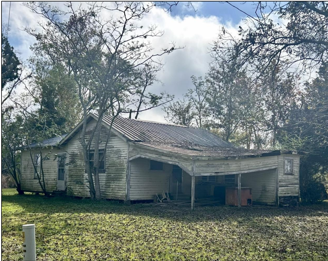
Figure 50. House at 1026 Ameda Berard, facing SE. (Resource No. 50-00802)
