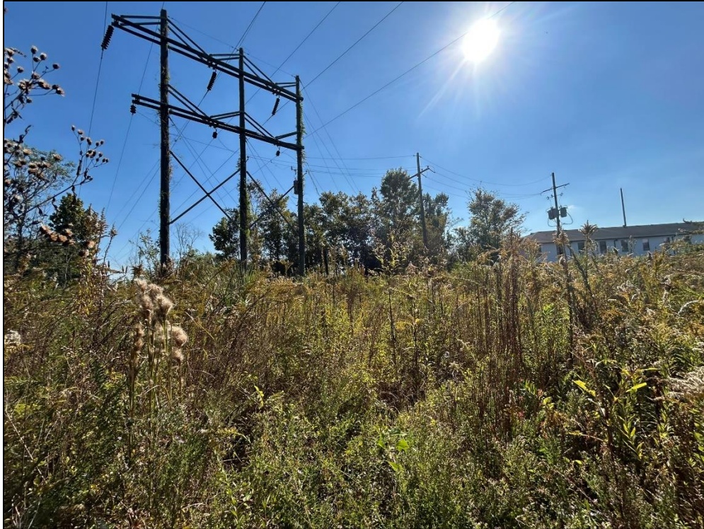
Figure 41. Powerline and brush within the northeastern portion of the APE, facing northwest.
