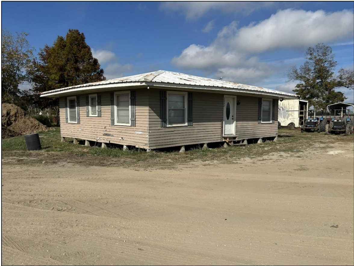
Figure 66. Building at 2842 Grand Point Hwy, facing northwest.
