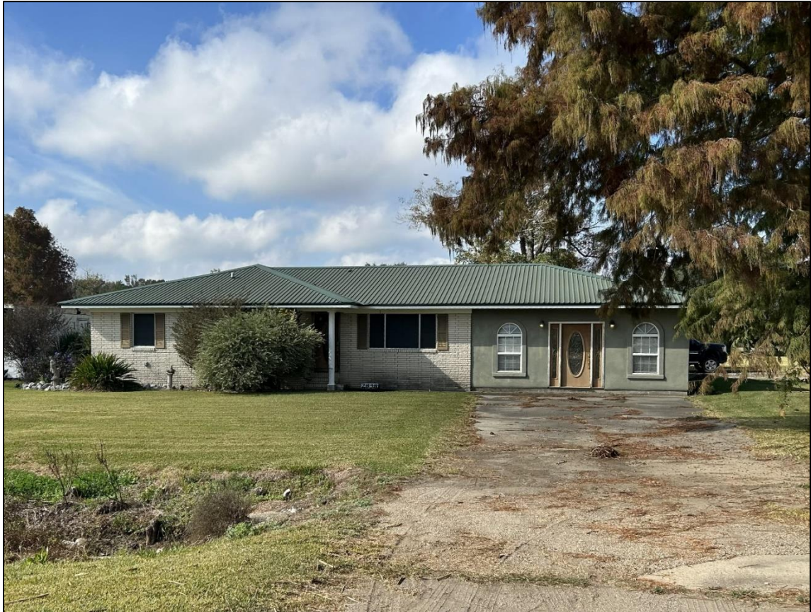
Figure 65. 2838 Grand Point Hwy, facing west.
