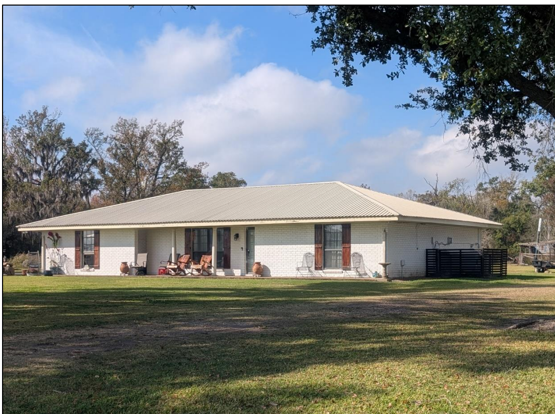
Figure 69. House at 2868 Grand Point Hwy, facing southwest.
