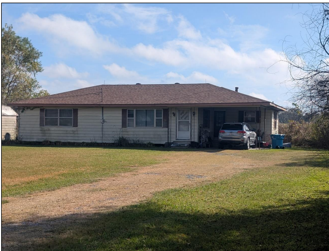
Figure 73. Structure at 2877 Grand Point Hwy, facing east-south-east.
