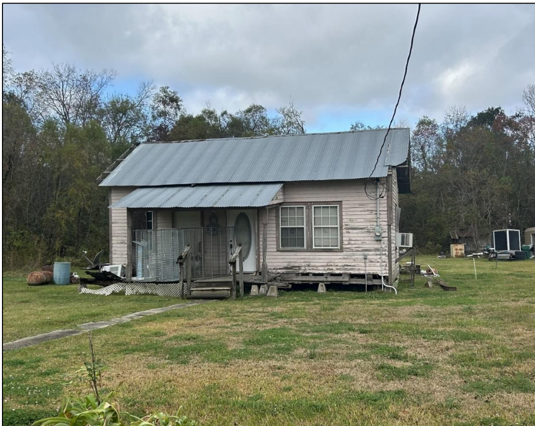
Figure 78. House at 1062 Paul Rd., facing south.
