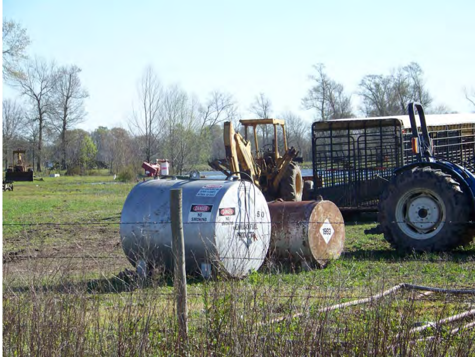
Photograph 19. Diesel fuel tanks with no secondary containment and agricultural equipment.
