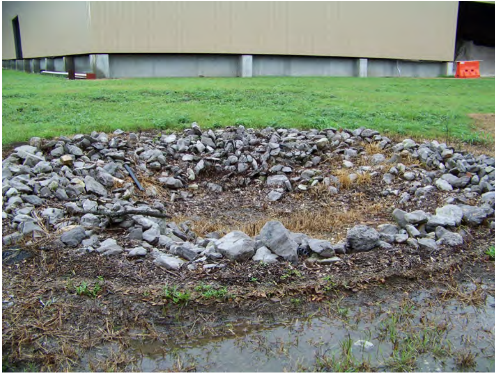
Photograph 9. Rock-Armored Storm Drain near Warehouse
