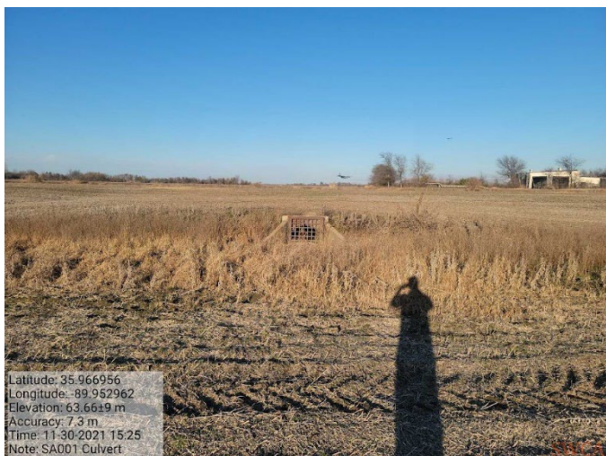
Photo C-5. Agricultural field drainage WCA001 connects to southern culvert (facing northeast).
