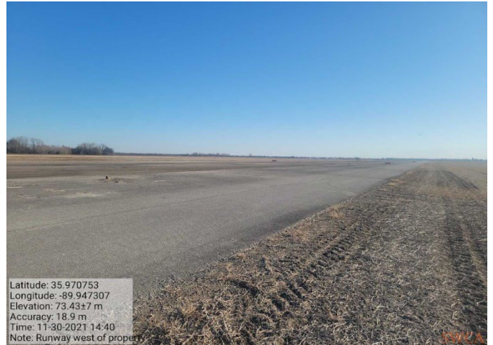
Photo C-10. Active runway in southwest portion of AOD.
