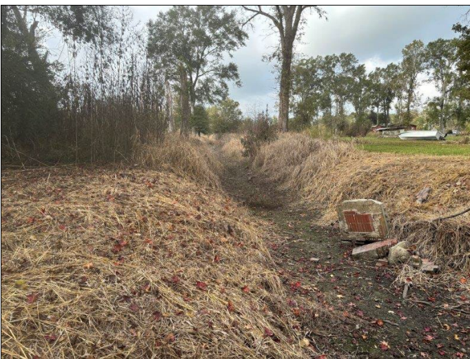
5. Drainage ditch along the northern property boundary
