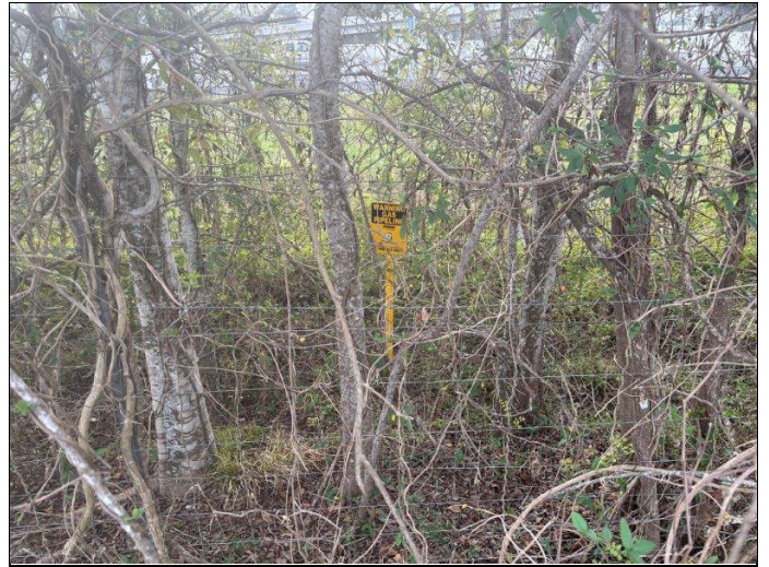
20. Natural gas pipeline marker
