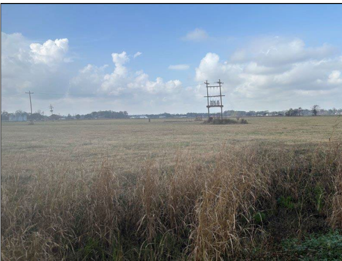
23. Electrical transformers and oil well west of the property
