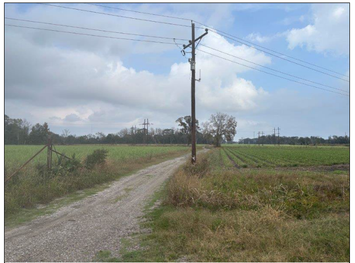
18. Gravel road facing north
