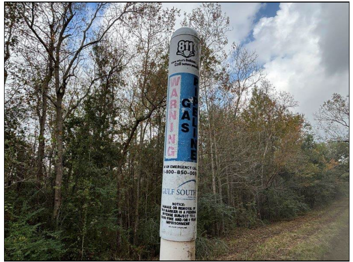
2. Gulf South Pipeline marker
