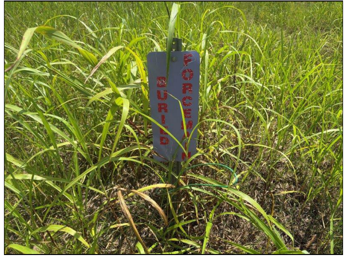
14. Buried force main marker
