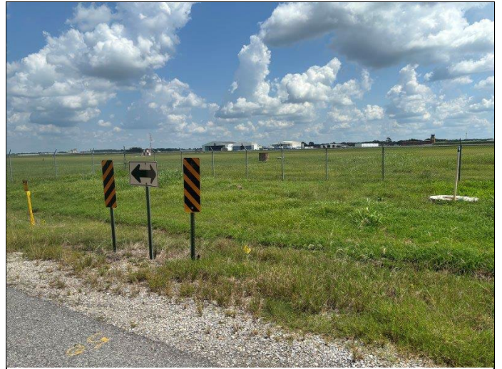
16. Northeast view toward the Acadiana Regional Airport
