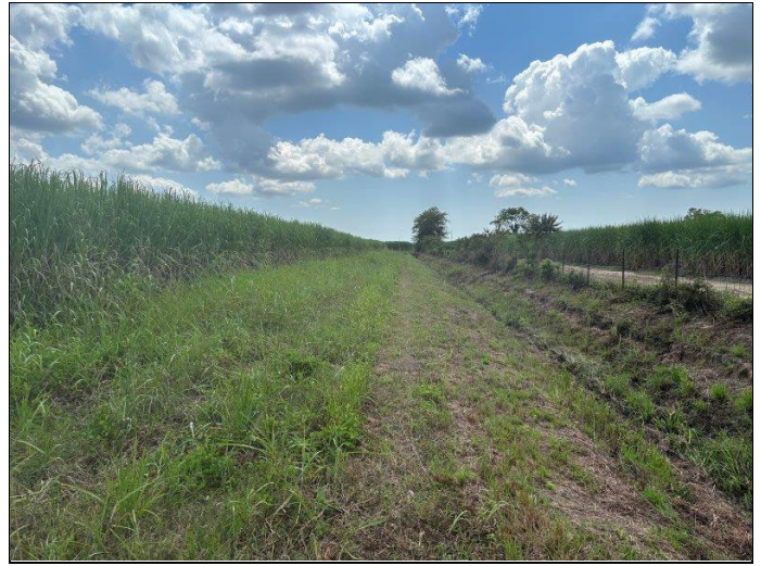
8. Southerly view of the western edge of the property along a sewer line right-of-way
