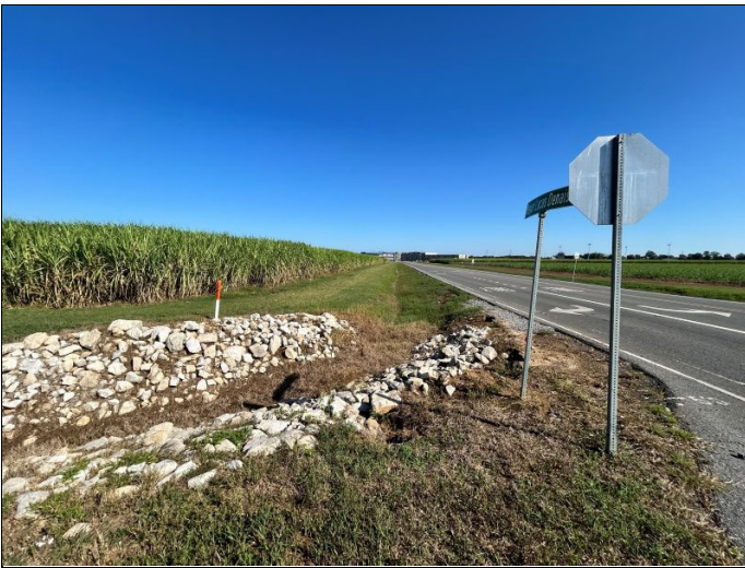
9. S3 – Roadside drainage ditch (along eastern boundary)
