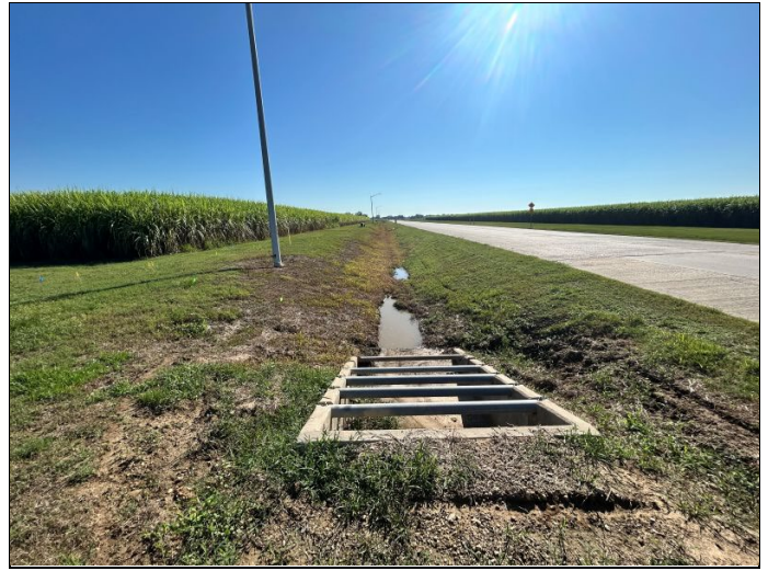
8. S3 – Roadside drainage ditch (along southern boundary)
