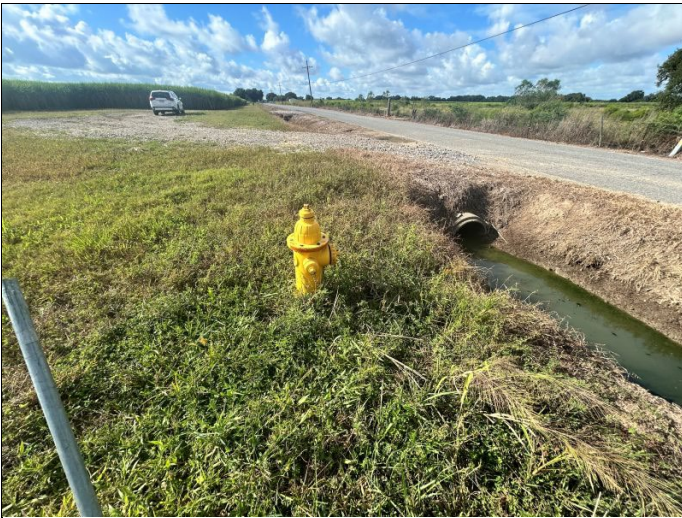
15. Representative fire hydrant and culvert on the subject property
