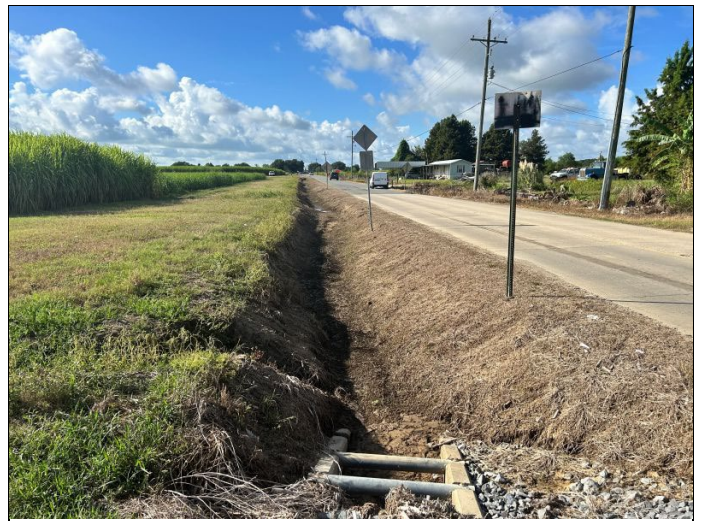
6. S1 – Roadside ditch on western boundary
