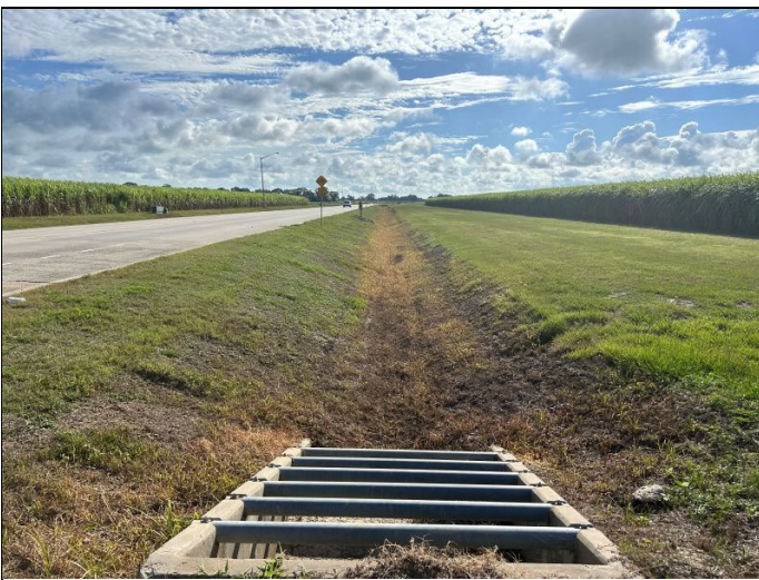
11. S6 – Roadside ditch on northern boundary
