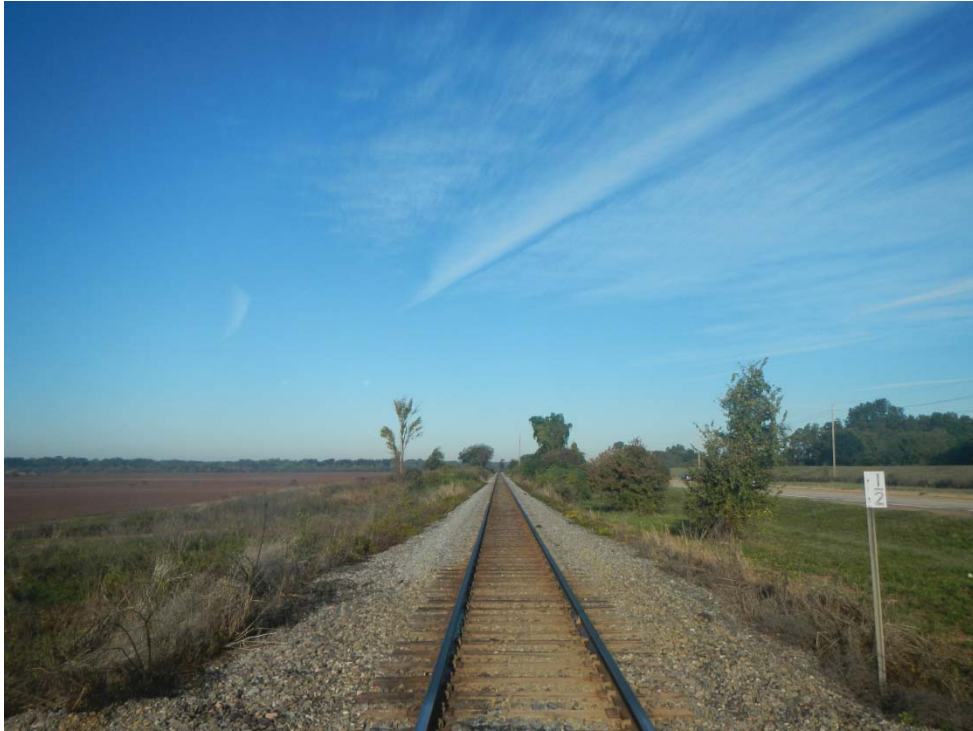
Train tracks run along the northeast border of the assessment property.
