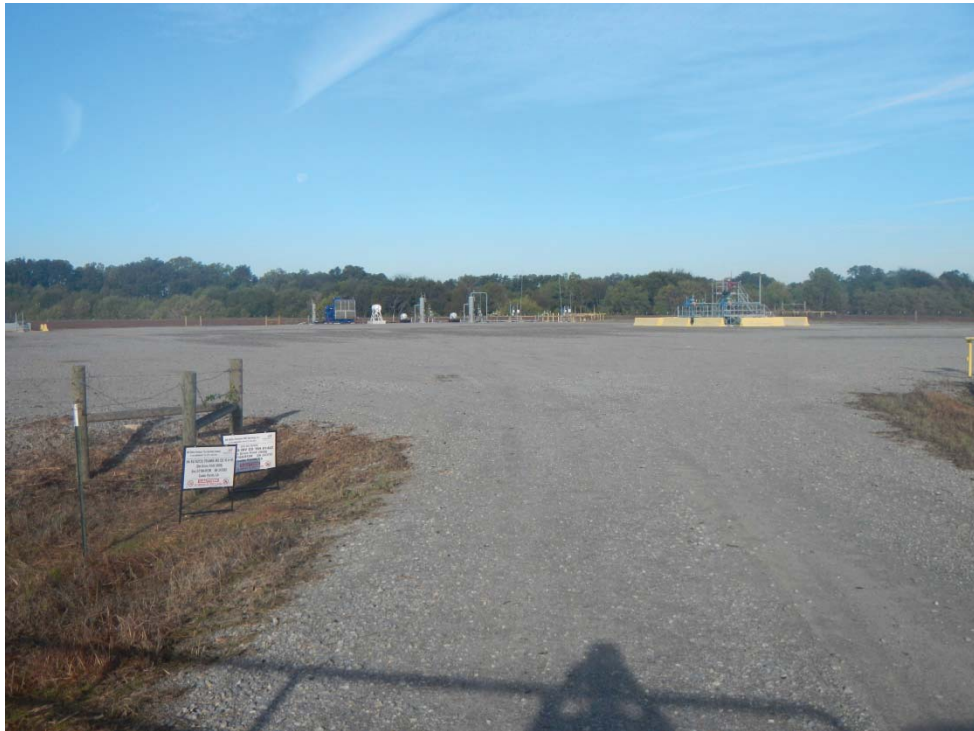
BHP Billiton Petroleum Company well site located near the northwest area of the assessment property.
