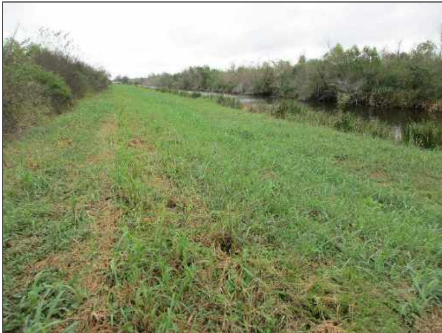
60 - Overview of levee and canal to the south, facing east.
