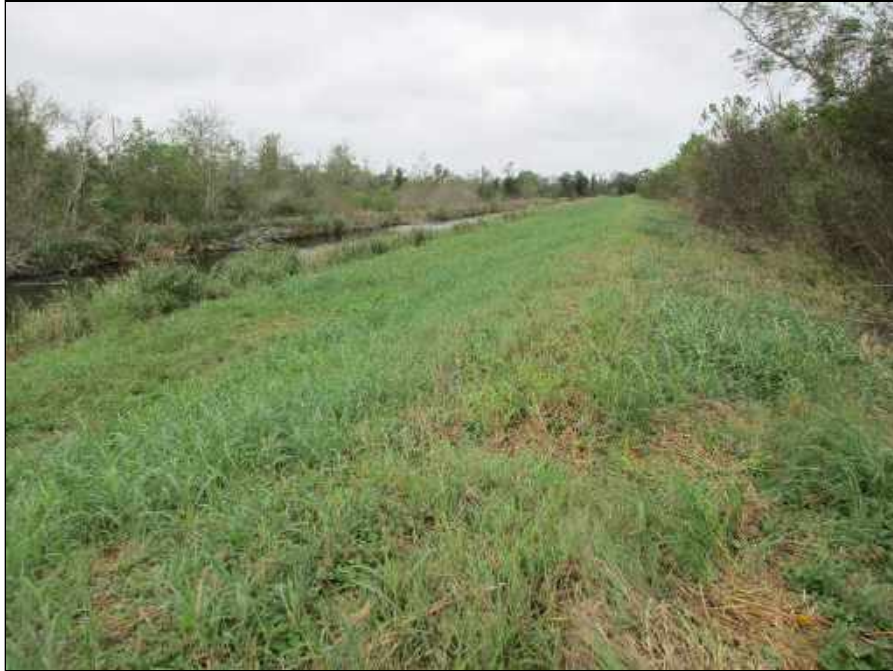
61 - Overview of levee and canal to the south, facing west.
