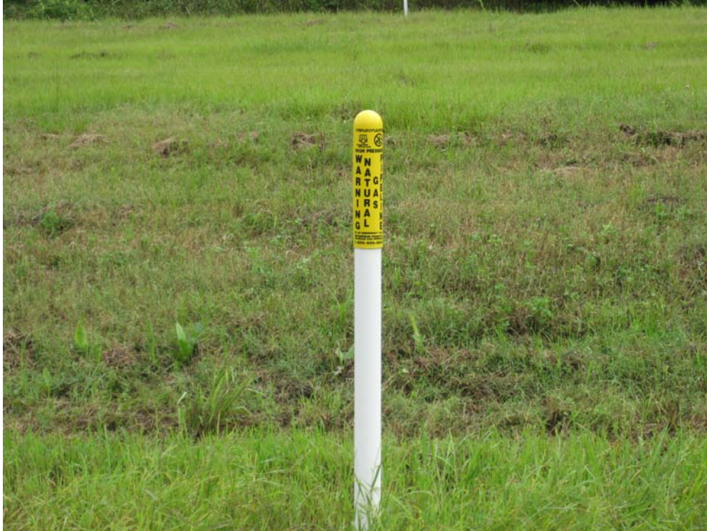
Photograph 13. Natural Gas Pipeline Marker
