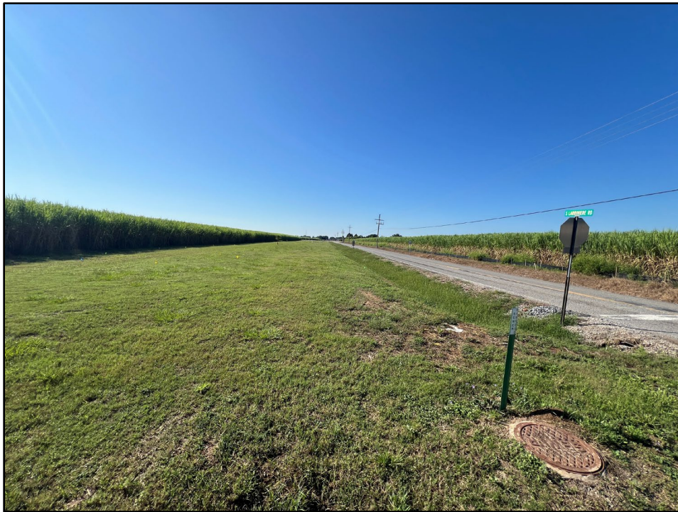
Photograph #11. NW corner of Subject property looking south. Pin flags marking below ground utilities and sewer manhole visible.
