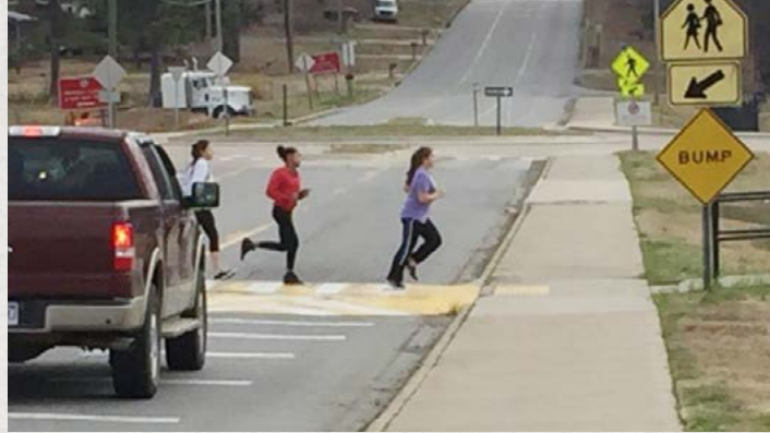
Raised crosswalks induce traffic to slow down, and are helpful for child safety near schools.
