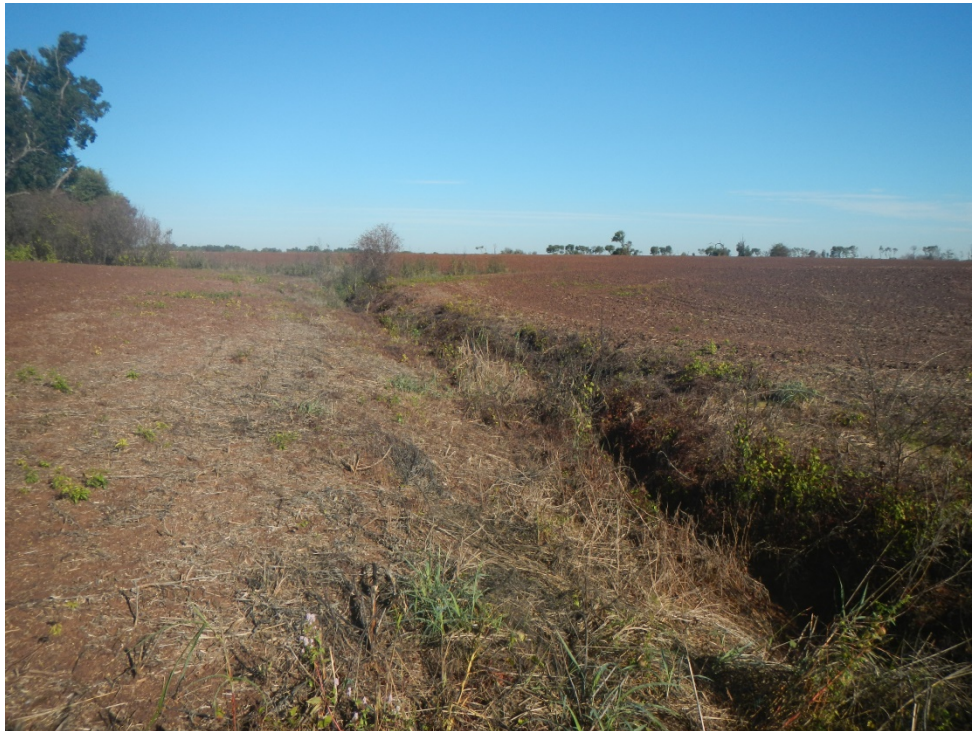
Drainage swale on the southern area of the assessment property.
