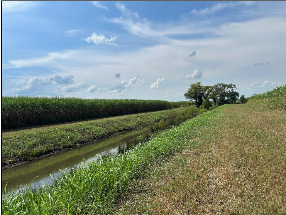
Figure 18. Right of way between crops, along canal, facing west.
