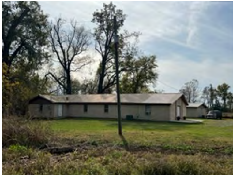
Baptist Church with transformer 1
