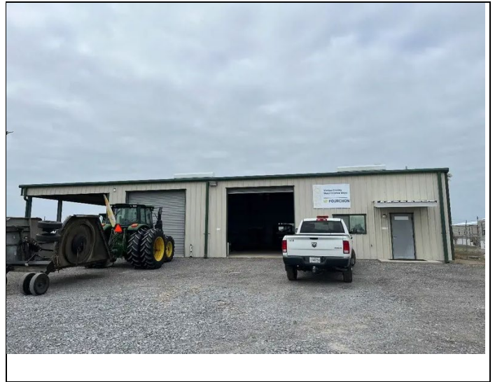
16. Maintenance building adjoining to the southeast corner
