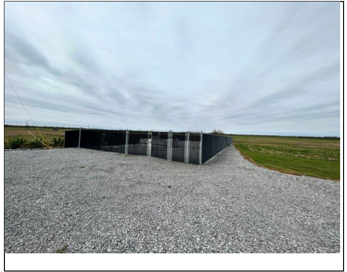
14. Wastewater treatment plant and sewer lift (southeast corner)
